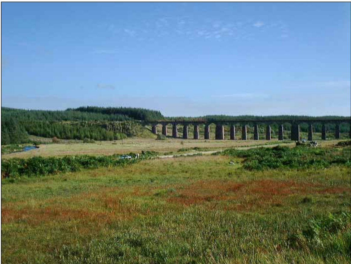
Big Water of Fleet Viaduct
